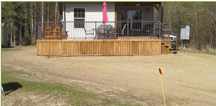
Figure 25. Example of sheathed in deck
