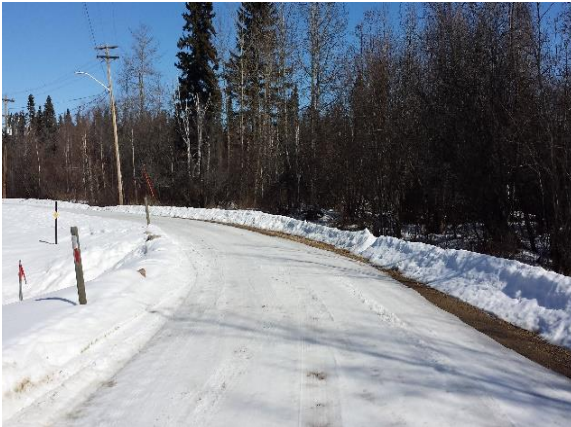
Photo 7: Crossing 1 overview; taken on March 20, 2019.
