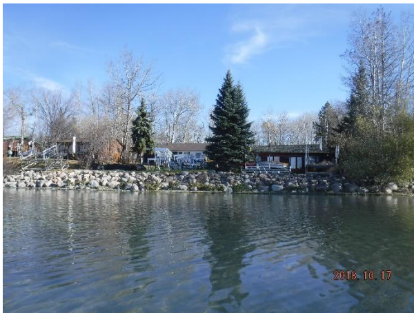
Photo 3: Shoreline disturbance including buildings, lawns, rock placement and vegetation clearing within Reach 2.
