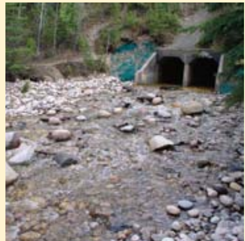
Canadian National Railway culvert after restoration.
