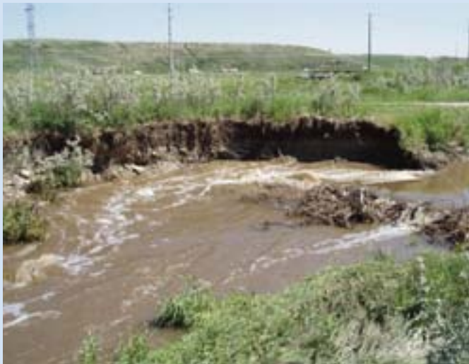
Erosion on West Nose Creek
